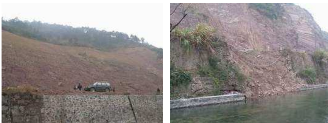
Fig. 2 Dragon's head mountain destroyed by Longhuguan landslide
