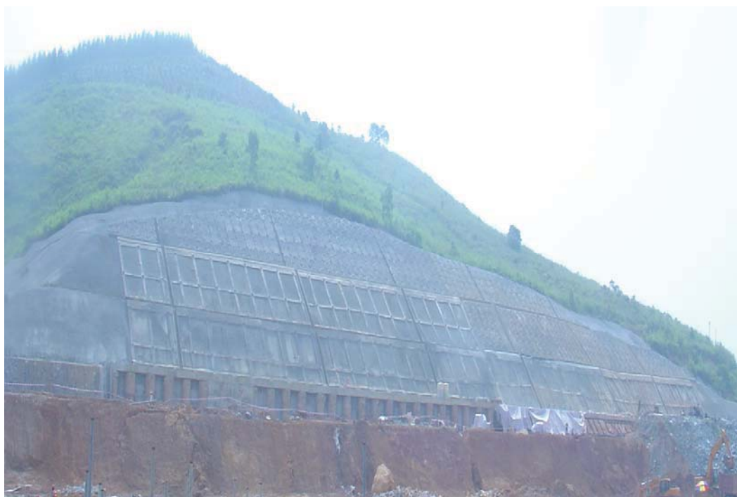
Figure 4 Reinforcement effect diagram of pressure dispersed anchor cable
