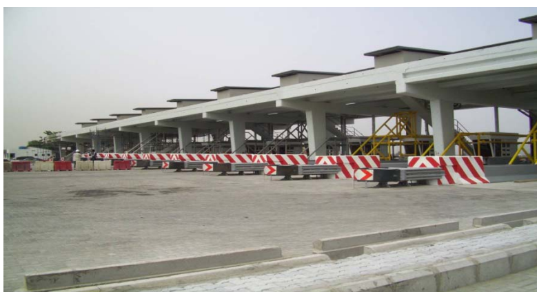
Figure 2 Admiralty Toll Plaza – Completed
