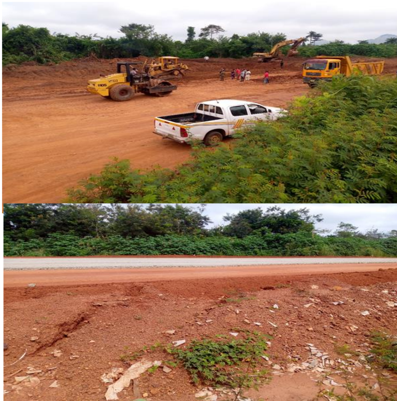
Fig. 2 Pictures showing the investigated Highway during the reconstruction/rehabilitation
